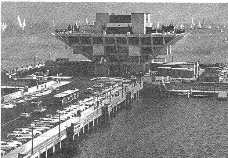
THE PIER — This new five-story inverted-pyramid building in St. Petersburg is just a part of the ocean-side complex at the new Feast site. The Pier includes two restaurants and a cocktail lounge on the fourth floor. There are also snack bars, meeting rooms, auditorium and exhibition areas, gift shops, an observation deck, plus a two-story fountain and fishing piers. [Photo courtesy St. Petersburg City News Bureau]
