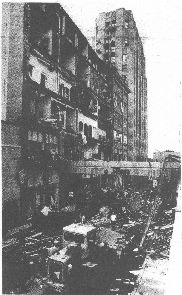
TORNADO AFTERMATH — Kalamazoo, Mich., residents clean up following May 13 storms and tornado. Two persons died in or just outside the devastated department store as winds ripped through the building. Many members reported instances of divine protection while nearby buildings and structures suffered extensive damage. [Photo by Rick Campbell, courtesy of the Kalamazoo Gazette.]
