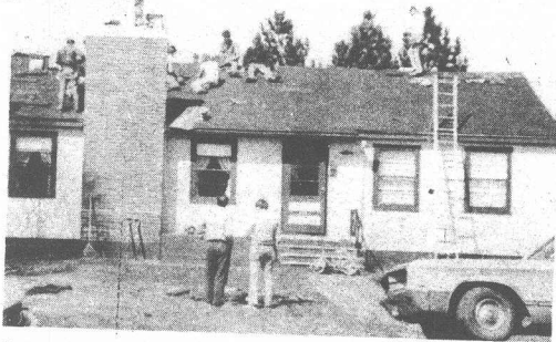
PATCHWORK — Duluth, Minn., members help repair the roof of the 27-year-old home of the Morkens April 27. (See "Church Activities," this page.)
