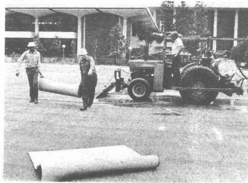
GREENER 'GRASS' — Workers remove the artificial grass Tartan surface from the infield of the Ambassador College track complex, worn through heavy use since the complex was built six years ago. Ambassador plant engineer Paul Troike said the track will be resurfaced with AstroTurf. [Photo by Roland Rees]
